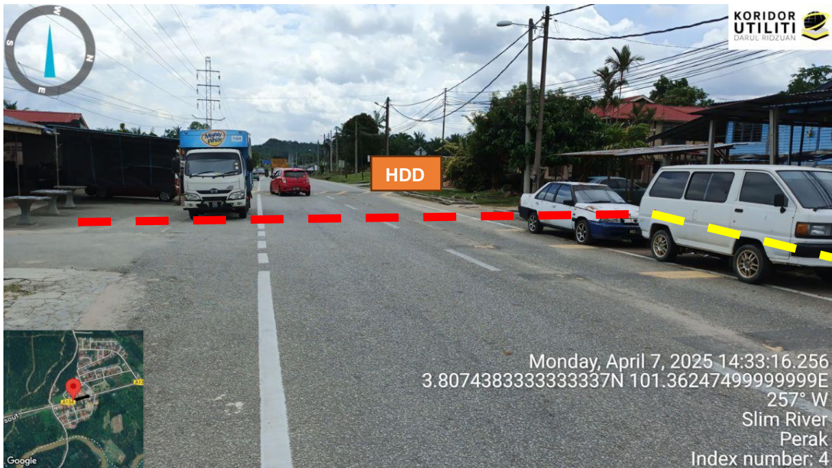
Rajah 4: Crossing Jalan Felda Besout – Kuala Slim
