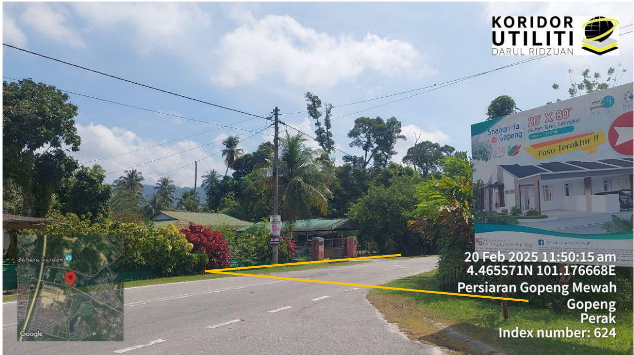
CONCRETE POLE 9 METER/EXTENSION POLE DI KAWASAN CROSSING OVERHEAD
