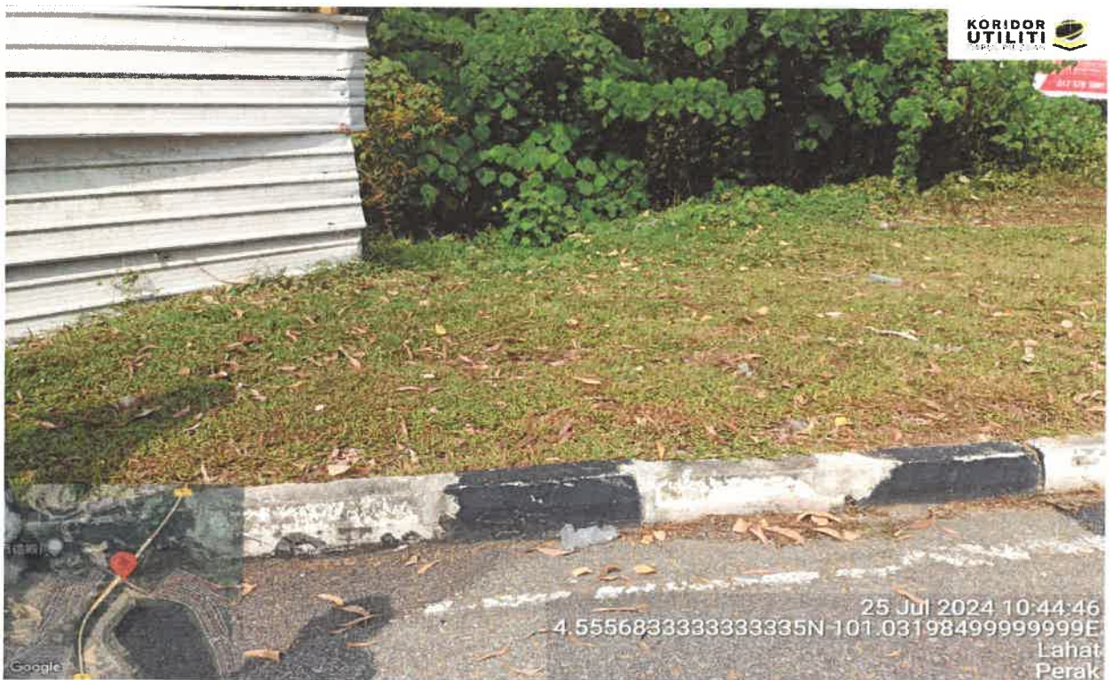
Lokasi Manhole baru (1) – Persiaran Lahat Mines
