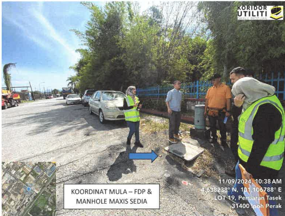
FDP & MANHOLE MAXIS – JALAN PORTLAND, TASEK
