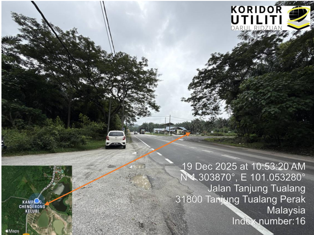
KAEDAH HDD BAGI JOINT PIT (CROSSING)
