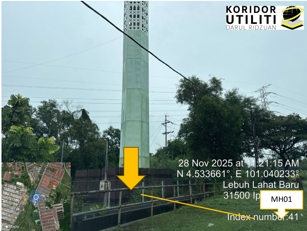
MICROTRENCHING 17 METER DAR MANHOLE CADANGAN
