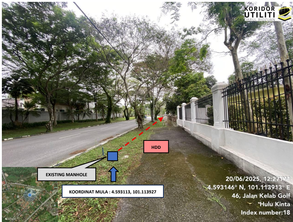
LOKASI KOORDINAT MULA KERJA HDD DI JALAN KELAB GOLF (Tapping from existing Maxis manhole)
