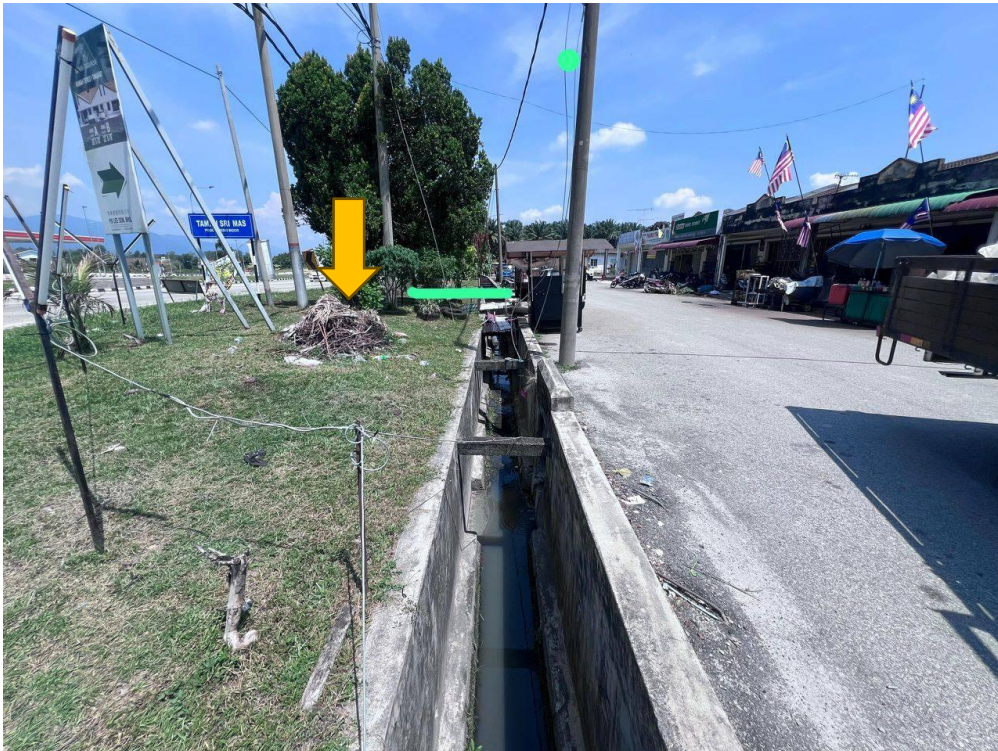
TAPPING EXISTING CABLE UNDERGROUND
