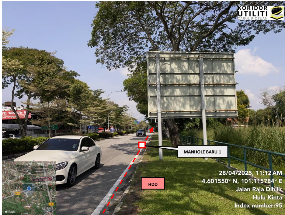
JAJARAN KERJA HDD DI JALAN RAJA DIHILIR (LOKASI MANHOLE BARU 1)
