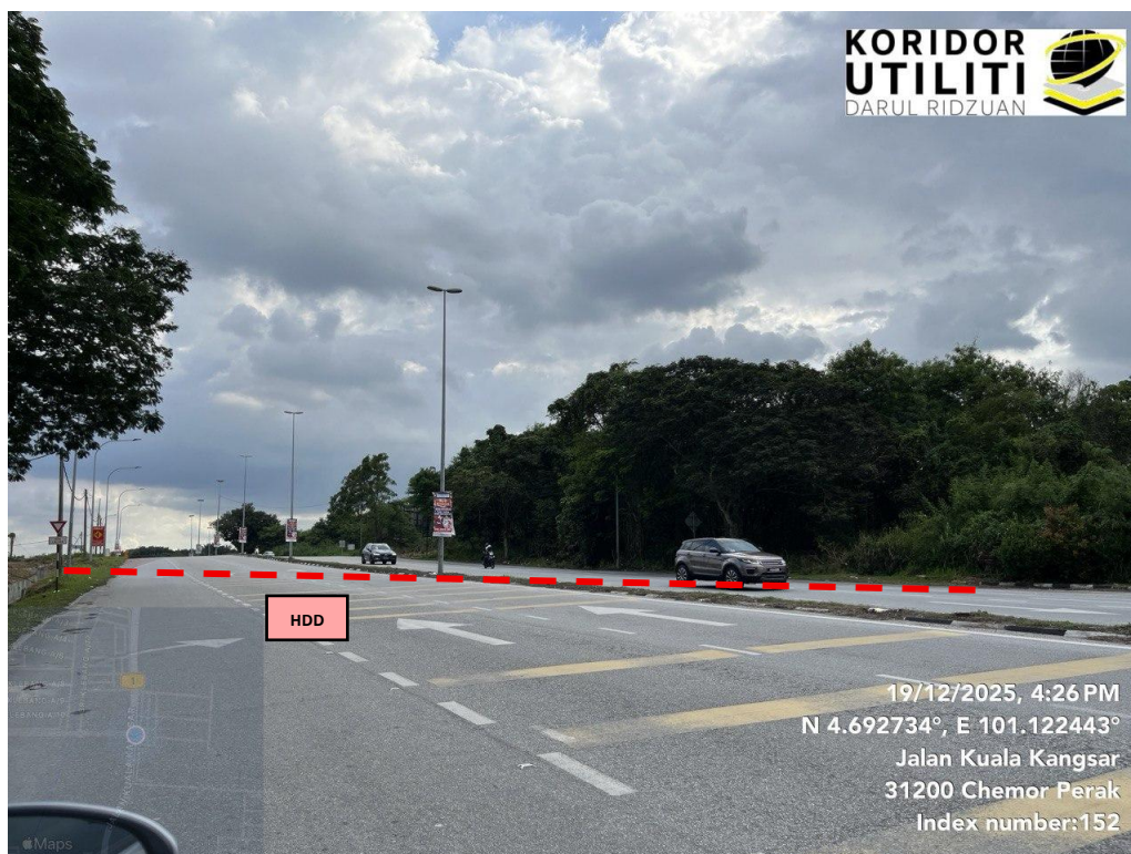
CROSSING HDD DI HADAPAN BHP JALAN KUALA KANGSAR
