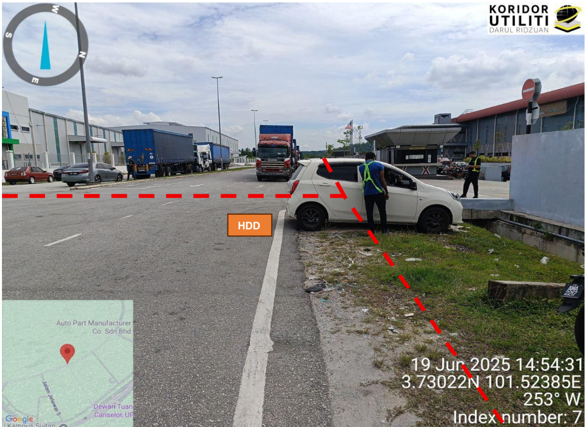
Rajah 11: Crossing Jalan Jelawai
