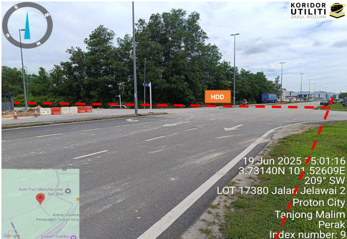
Rajah 10: Crossing Jalan Jelawai
