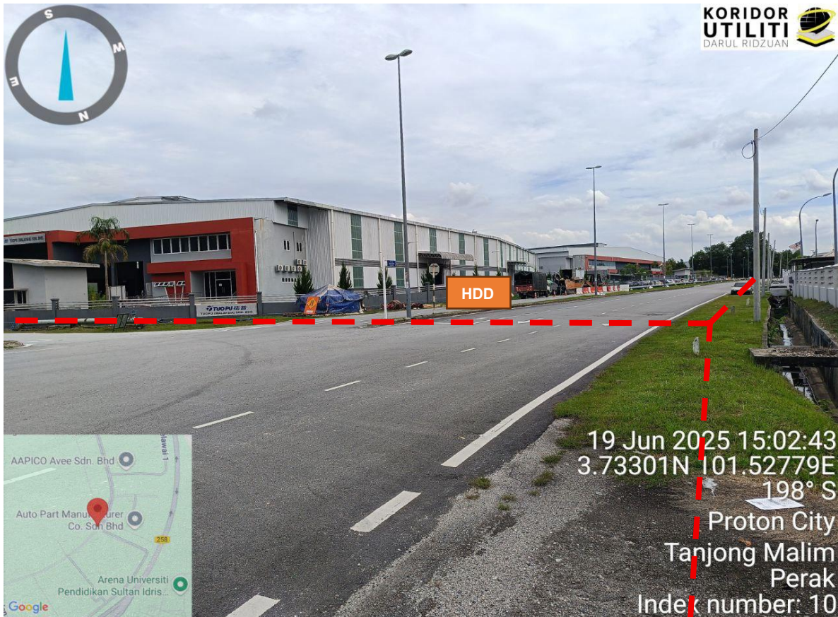
Rajah 9: Crossing Jalan Jelawai
