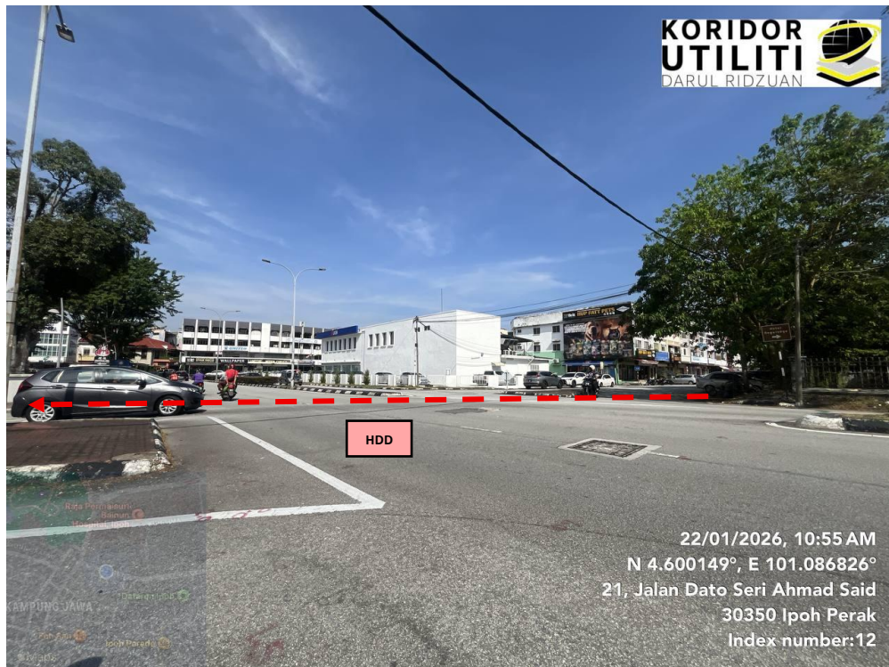
JAJARAN KERJA HDD DI JALAN DATO SERI AHMAD SAID
