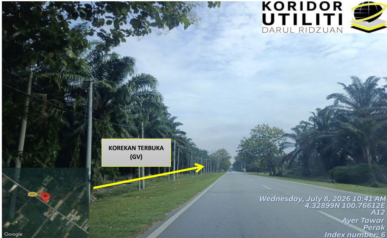
JALAN TRANSDINDING, AYER TAWAR (A12)
