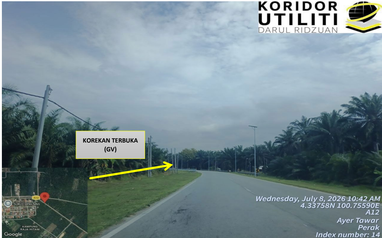
JALAN TRANSDINDING, AYER TAWAR (A12)
