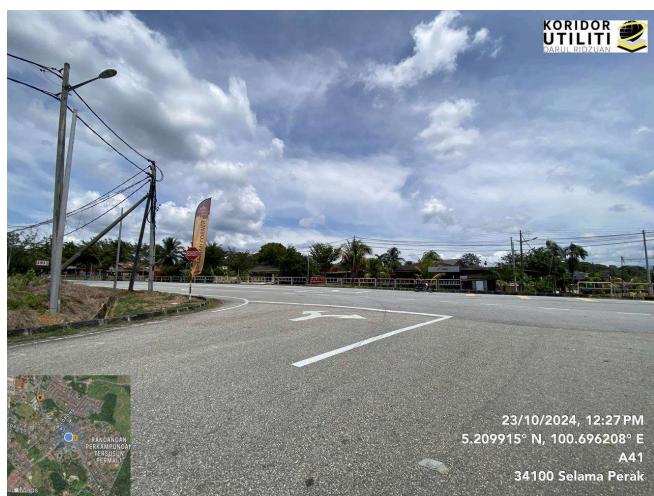
Laluan kaedah Pipe Jacking
