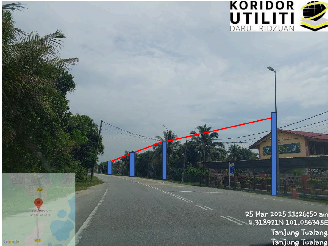
JAJARAN PENANAMAN TIANG DI JALAN PUSING – TG TUALANG (A15)
