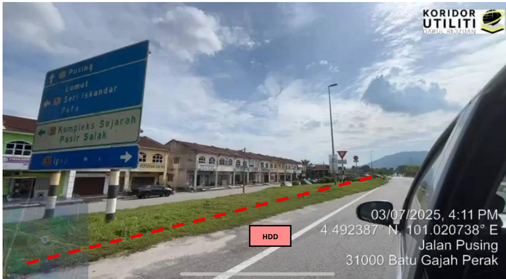
JAJARAN KERJA HDD DI JALAN PUSING – TG TUALANG (A15)
