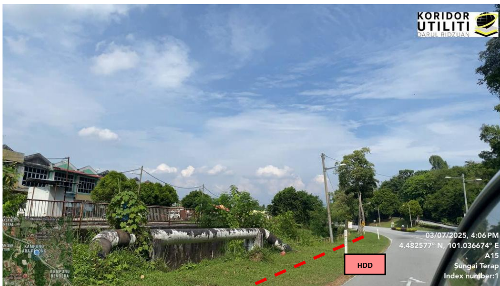
JAJARAN KERJA HDD DI JALAN PUSING – TG TUALANG (A15)
