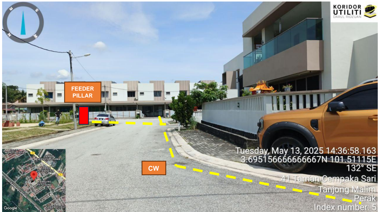
Rajah 5: Crossing di Jalan Pelangi 6 ke Feeder Pillar
