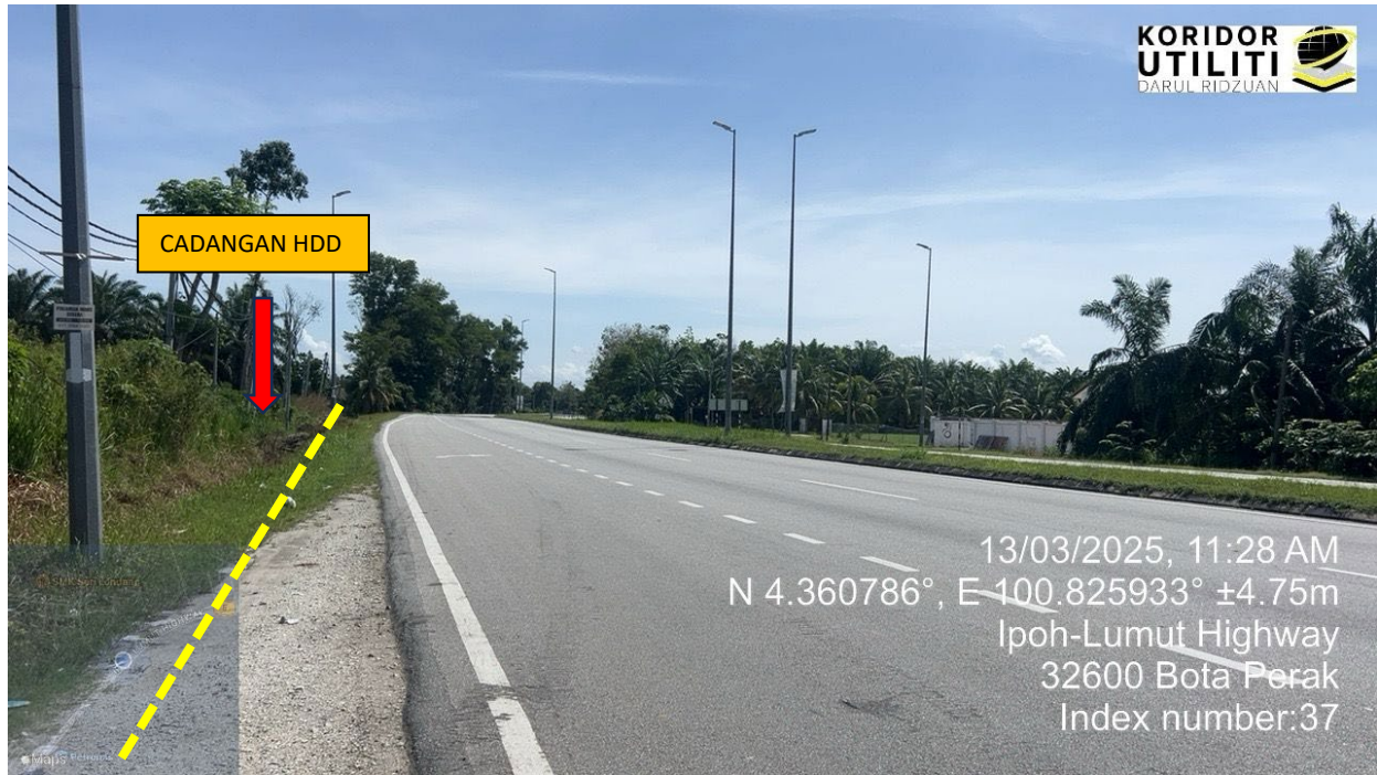
GAMBAR 4: JALAN LUMUT – IPOH KAEDAH HDD
