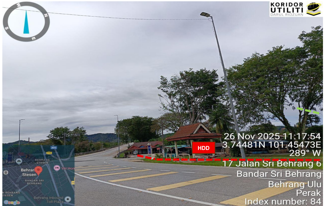
Rajah 7: A124 Jalan Behrang Stesen – Jalan Sri Behrang 4
