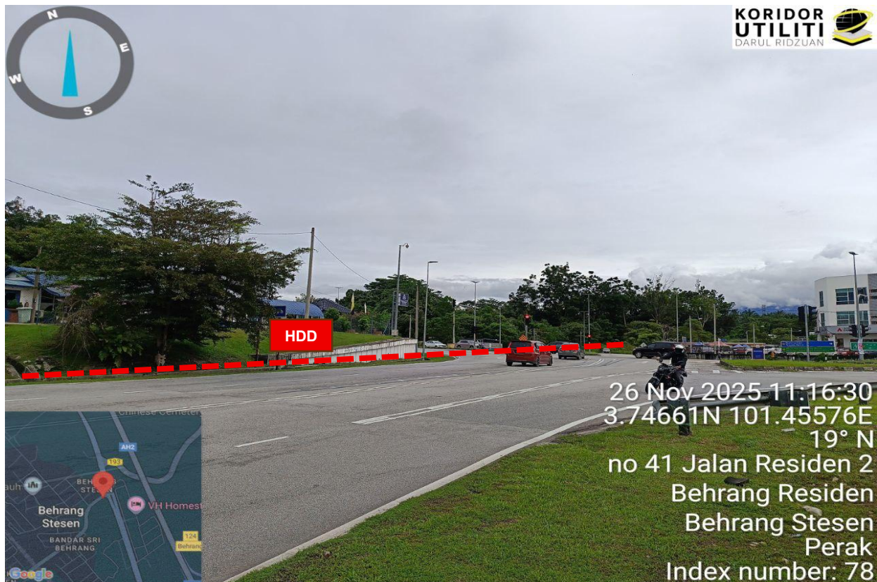
Rajah 4: A124 Jalan Behrang Stesen
