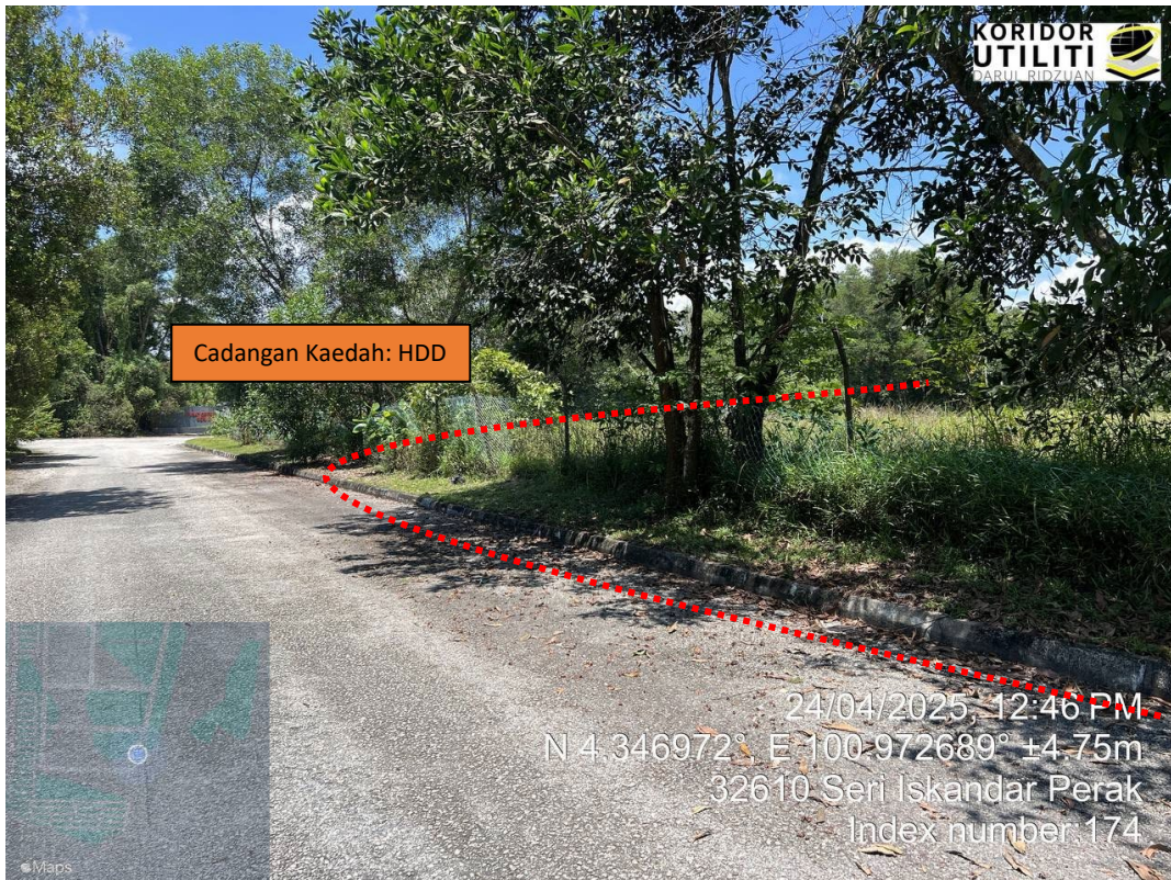
LOKASI KERJA: JALAN TEKNOLOGI 9 KE ARAH NORTHERN CENTRALIZED INJECTION STATION (KAEDAH HDD)
